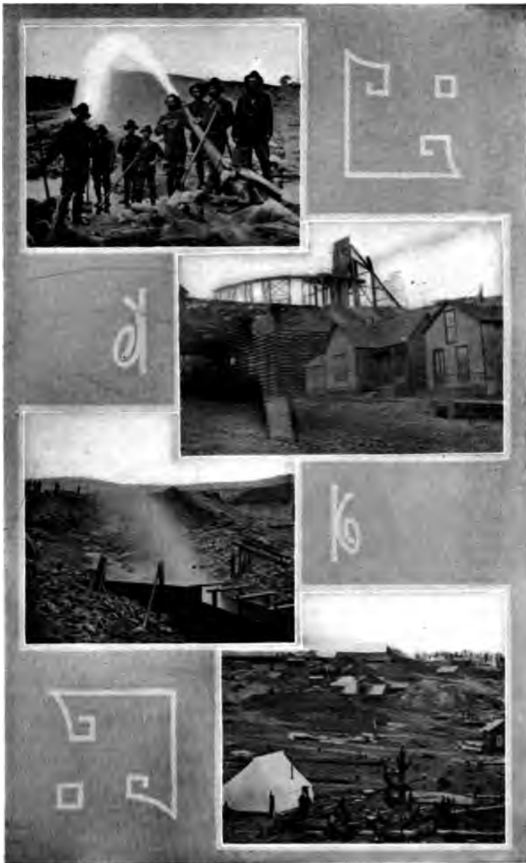
HYDRAULIC MINING Breaking down the Banks in California Gulch
